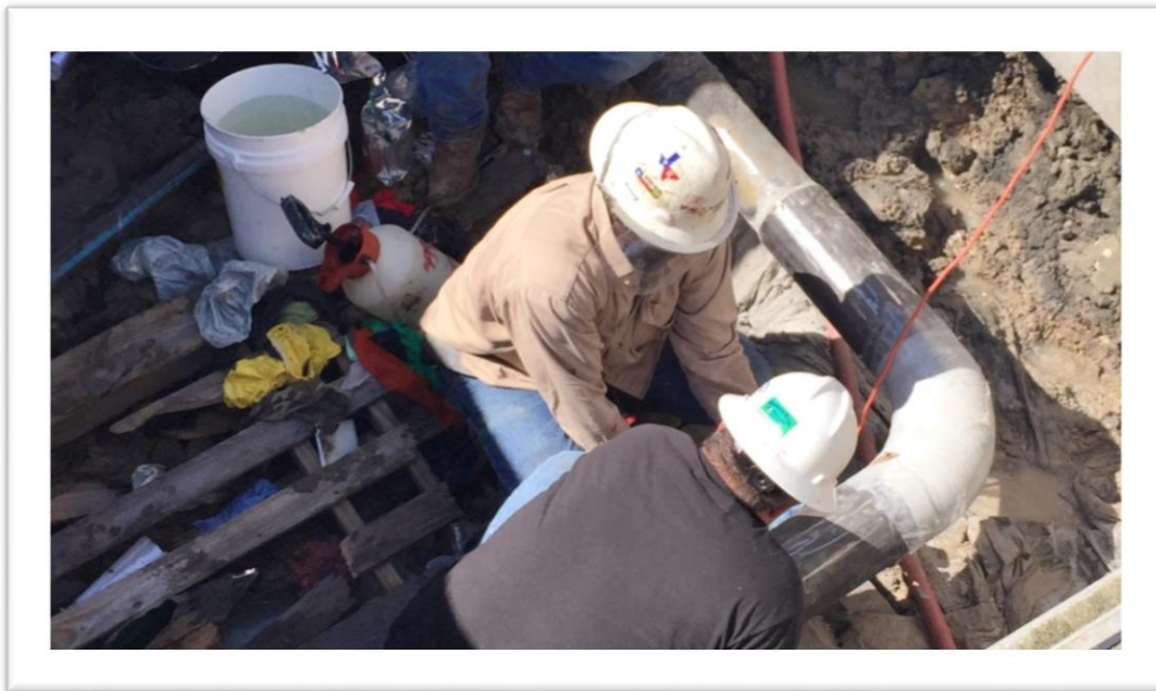
Finishing-off with the patented composite wrap.
