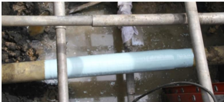
Finished process and ready for backfill.
