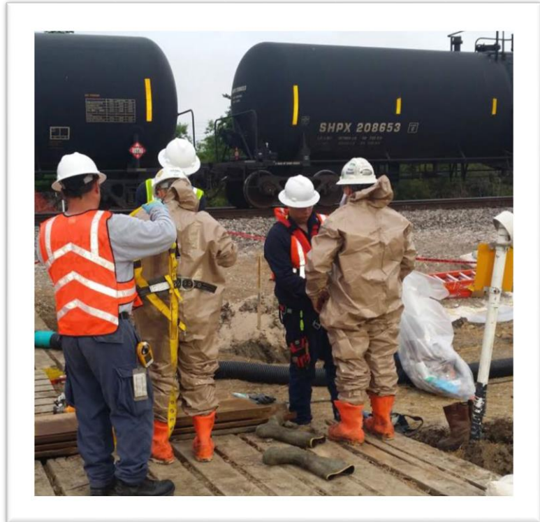
Contract personnel preparing to enter the excavation and make necessary repairs.
